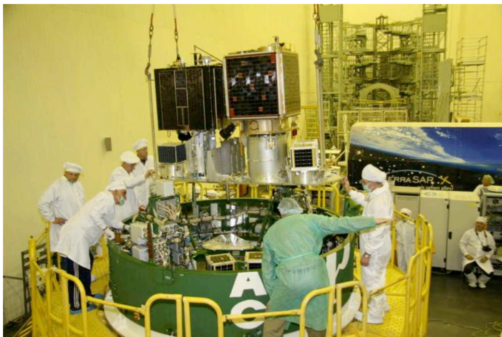
Figure 3: Integrated Payloads being loaded into the Dnepr 2007 cluster launch
