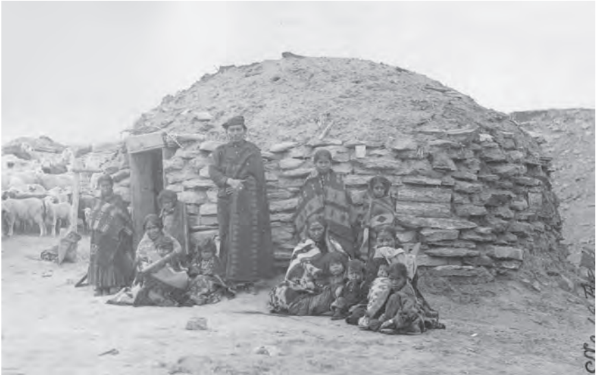
A family in front of their stone hogan. Evans believed that the Navajos borrowed design elements of this structure from the Pueblo Indians. Photo by William Pennington.
