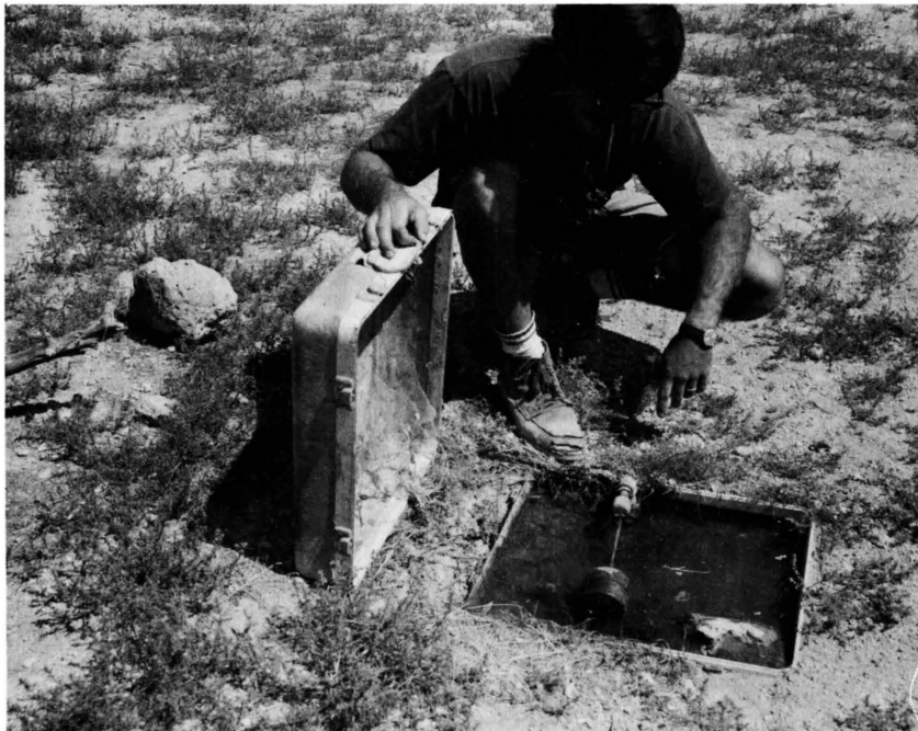
Figure 4. Drinking basin typical of those used in guzzlers on the Thomas and Dugway Mountains.
