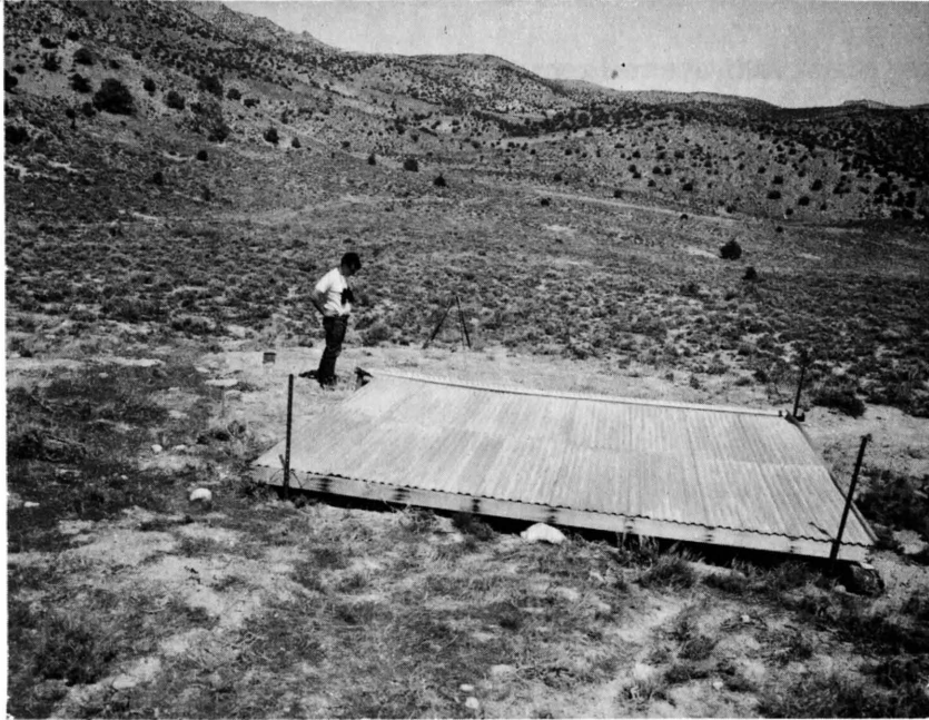
Figure 3. Metal rain-catchment apron used in guzzlers on the Thomas and Dugway Mountains.
