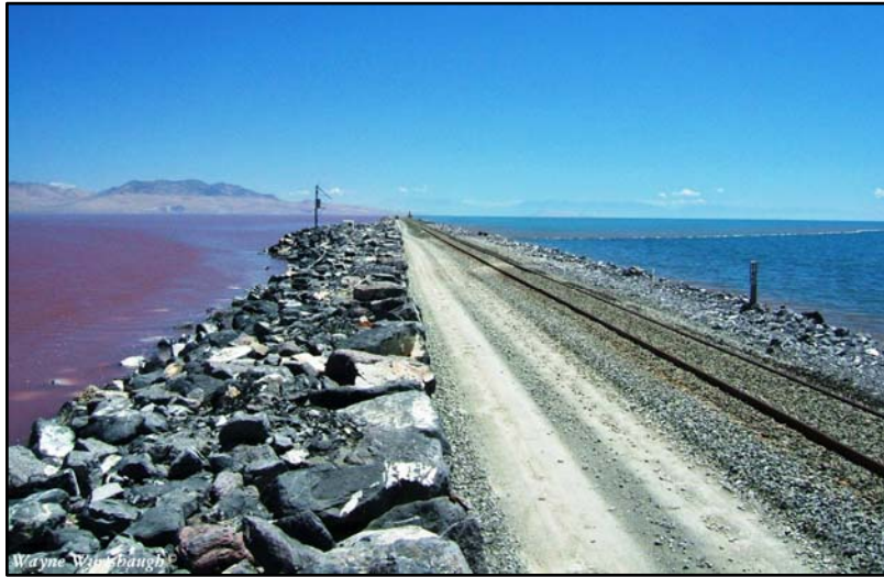
Fig. 22. The Southern Pacific Railway causeway separating Gunnison Bay (left) from Gilbert Bay (right).
