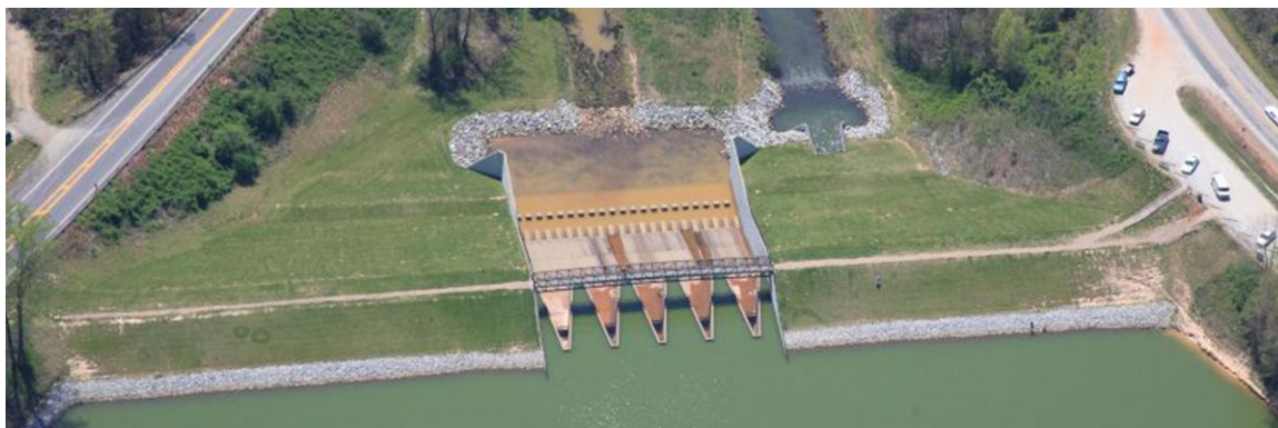
Fig. 2. Example of prototype labyrinth weir. (Yahoola Dam, Georgia. Photo courtesy of Schnabel Engineering)
