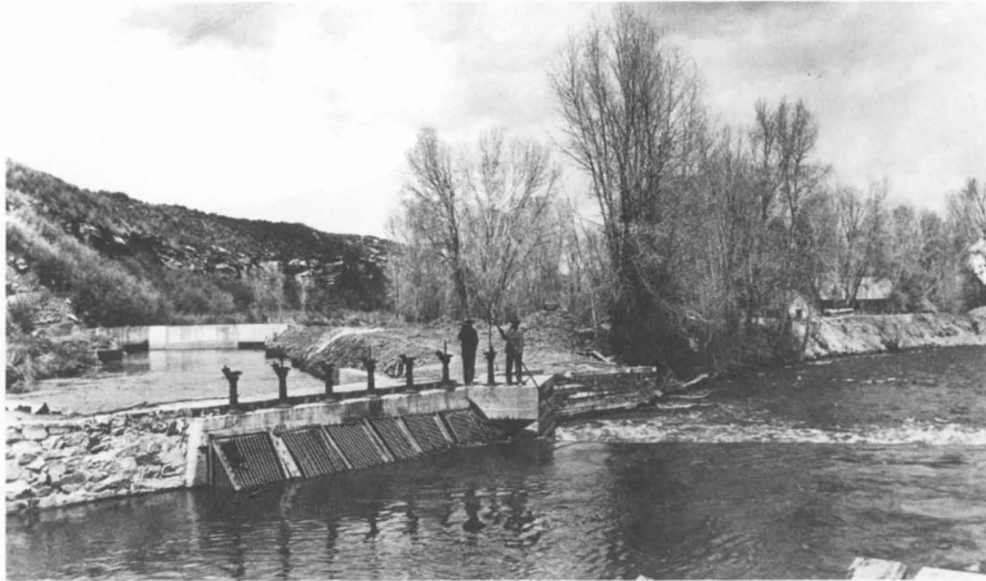
With maintenance costs for wooden equipment proving exorbitant, the Board of the Montezuma Valley Public Irrigation District decided to replace the deteriorated wooden headgates with concrete and steel ones in 1949. (Dolores Archeological Program Records, Dolores, Colorado)
