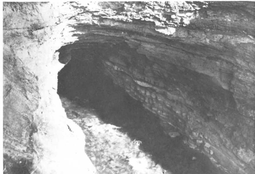
The Montezuma Valley Water Supply Company began this mile long tunnel in 1885 using Sergeant drills powered by air compressors. The tunnel was placed on a one percent grade and was built nine feet wide and seven feet high. (Dolores Archeological Program Records, Dolores, Colorado)
