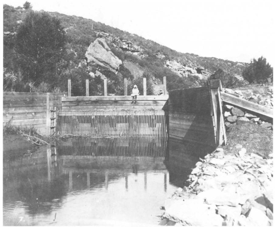
Originally all headgates of the irrigation system were built of wood like the one shown here. (Dolores Archeological Program Records, Dolores Colorado)
