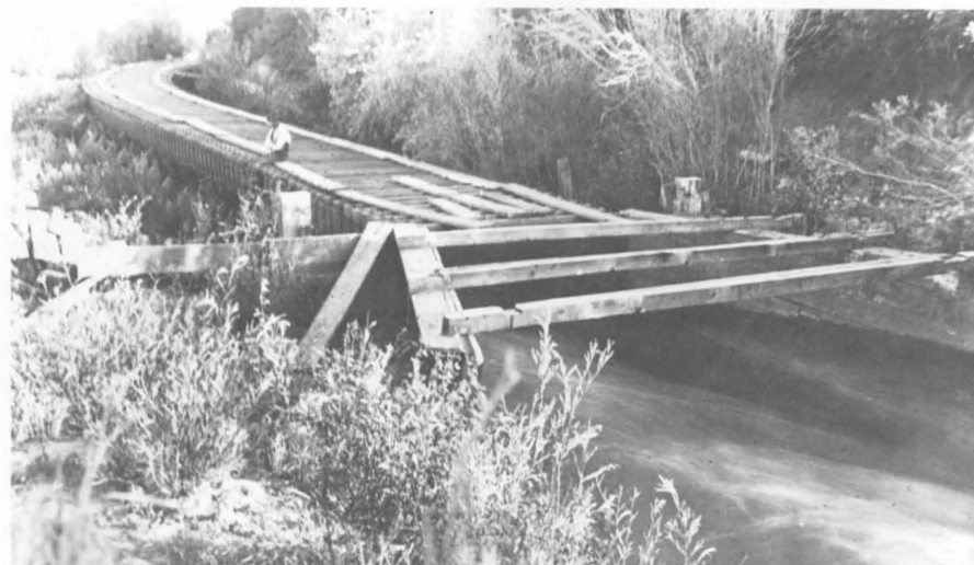
The Morton Flume, shown here in 1951, and the Dolores Number Two Canal carried the Dolores River water through a "Great Cut" across the divide to supply areas in the Montezuma Valley with irrigation. (Dolores Archeological Program Records, Dolores, Colorado.)
