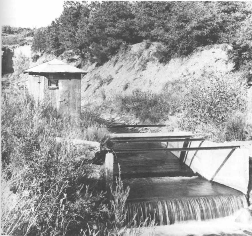
The irrigation system never attained the potential of its historic boosters such as James W. Hanna. Gauging Station along irrigation canal. (Jet Lowe, HAER)
