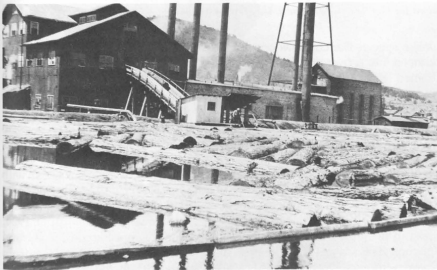
The mill pond was capable of holding one million board feet of logs. (Robert Orr Collection)
