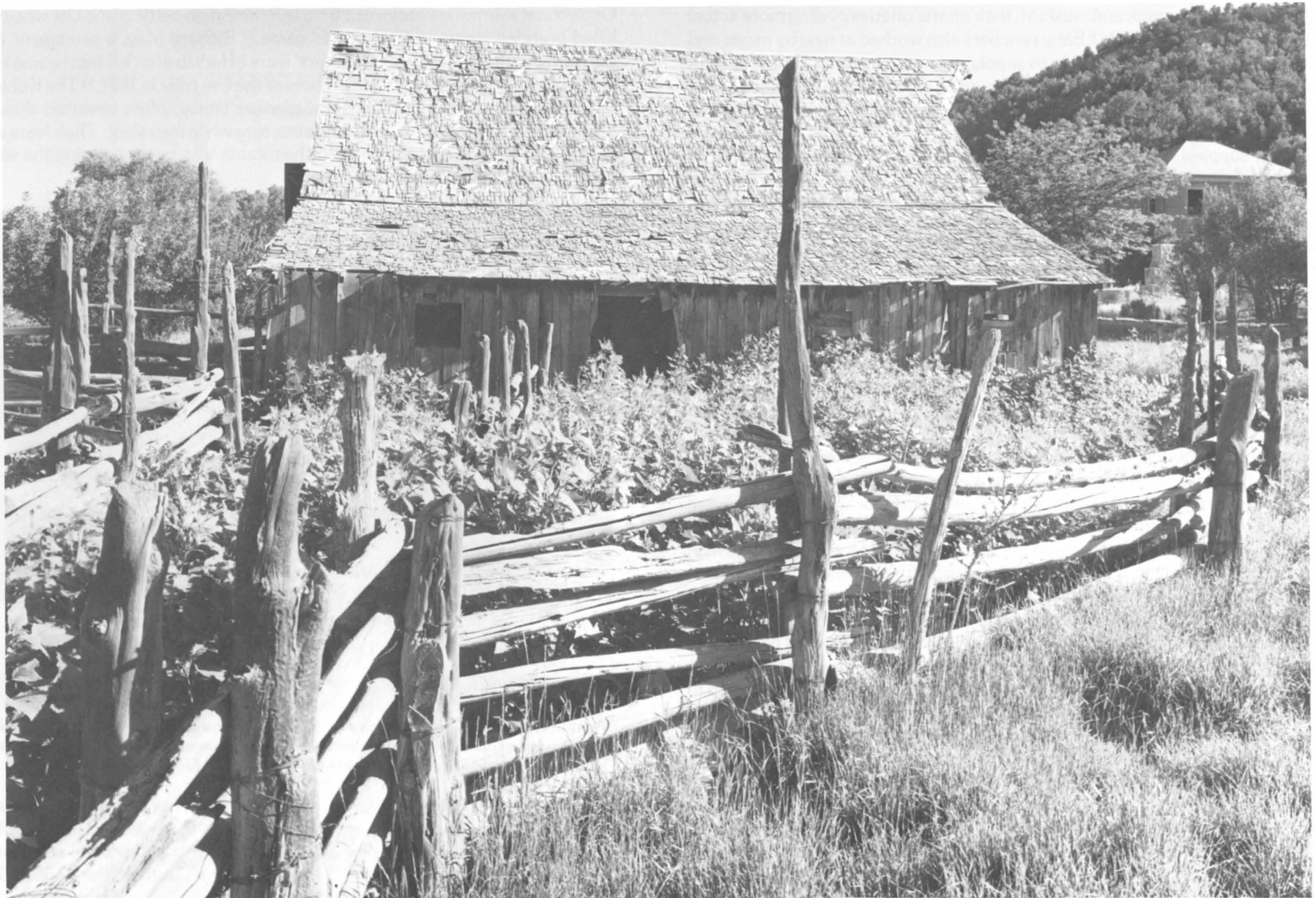
August Kuhlman died in 1926 and shortly thereafter the operation was purchased by Albert Seeger. The Periman brothers, Tillman and Reuben, acquired the property in 1932 and added dairy cows to their cattle herd. The cattle barn was typical of similar structures in the valley with its frame shed added later to the original log barn.
