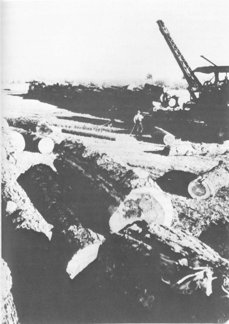
McPhee utilized narrow gauge railroads to assist in their logging. Mechanical loaders hauled the cut timber onto flat railroad cars. (C.W. Sward, U.S. Forest Service)
