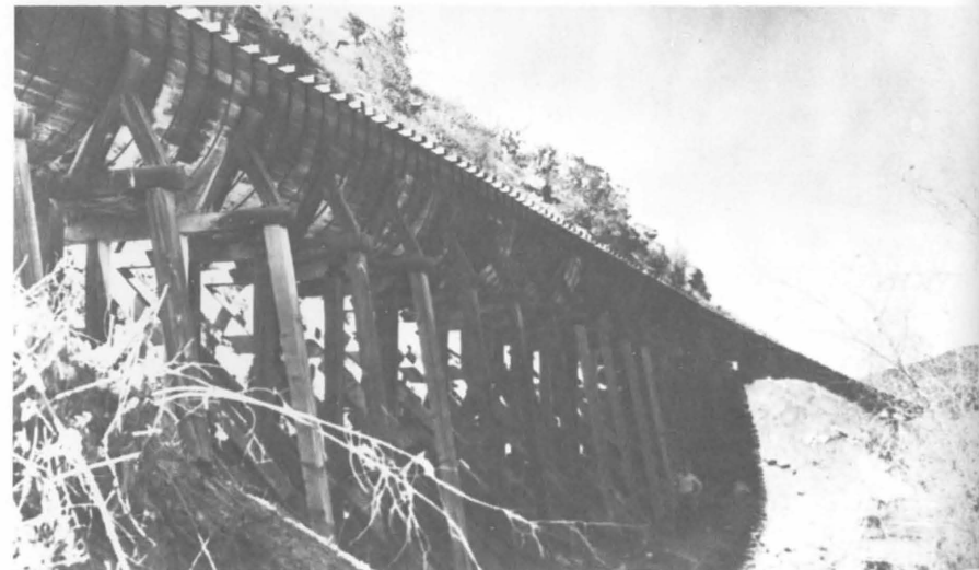
The wooden Morton flume had unusually large dimensions, measuring 18 feet wide, seven feet deep and 5,850 feet long. (Dolores Archeological Program Records, Dolores, Colorado)
