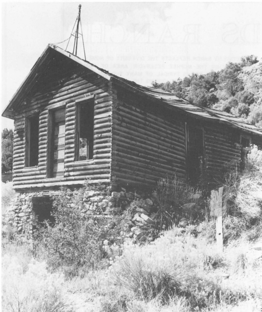
The lumber used in the construction of Reynolds home was given to him in lieu of back wages from the lumber company at McPhee. (Jet Lowe, HAER)
