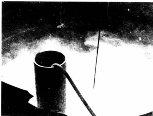
Figure 14.—Aeration tank surface. Photo P801-D-80760.
