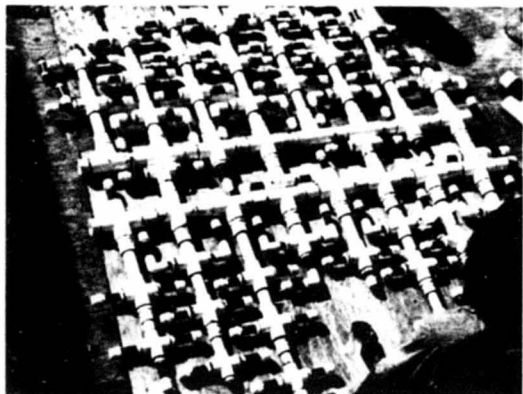
Figure 12 - Diffuser pipe network. Photo PB01-D-80759.
