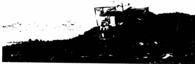
Figure 3.3-9. Earthen-mound islands can easily be constructed with a bulldozer during impoundment construction (Jones 1975).
