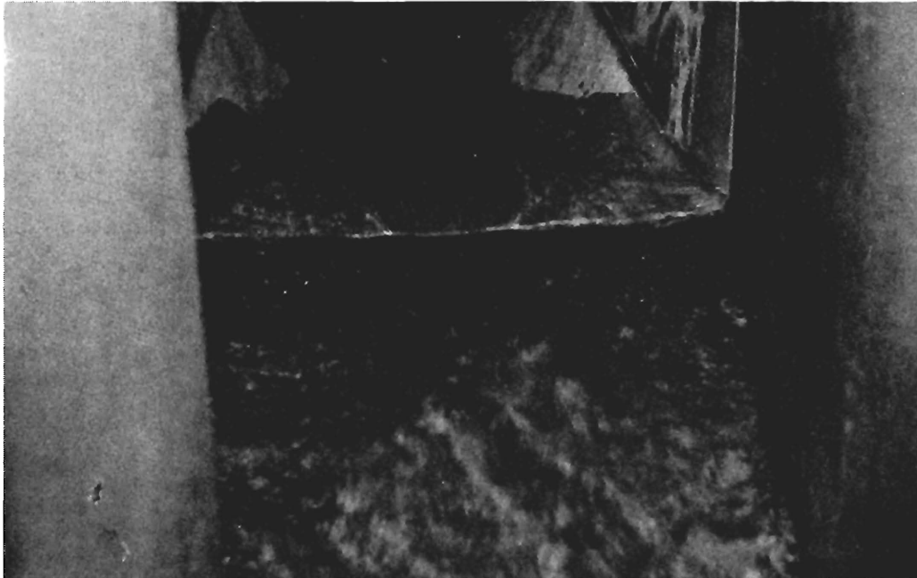
Figure 18. Typical view of low flow in the entrance section of the 18-inch Parshall flume. (Free flow, Q = 1 cfs, H_a = 0.191 ft, the slope of the incoming concrete pipe = 0.0080, facing upstream.)
