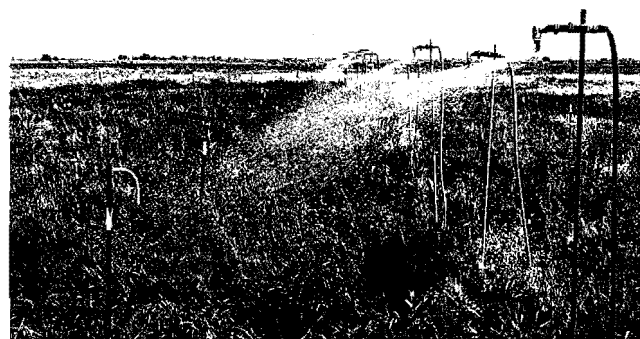
Figure 3. Wastewater application sprinklers for the overland flow system.
