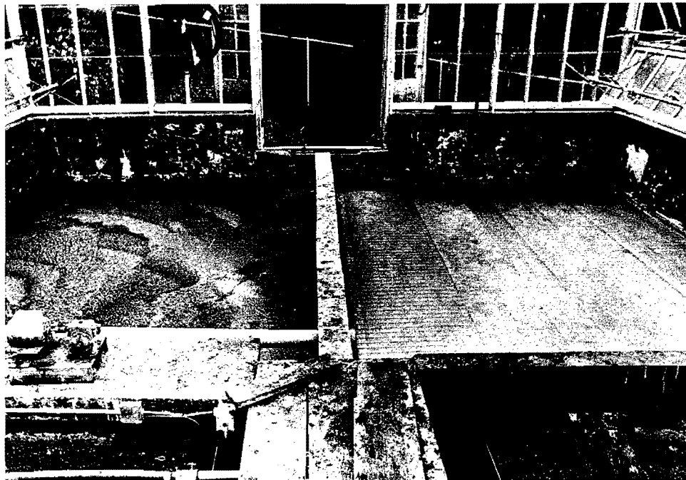
Figure 6. Wedgewater filter bed sandbed conversion, Clarks Green, Pennsylvania.
