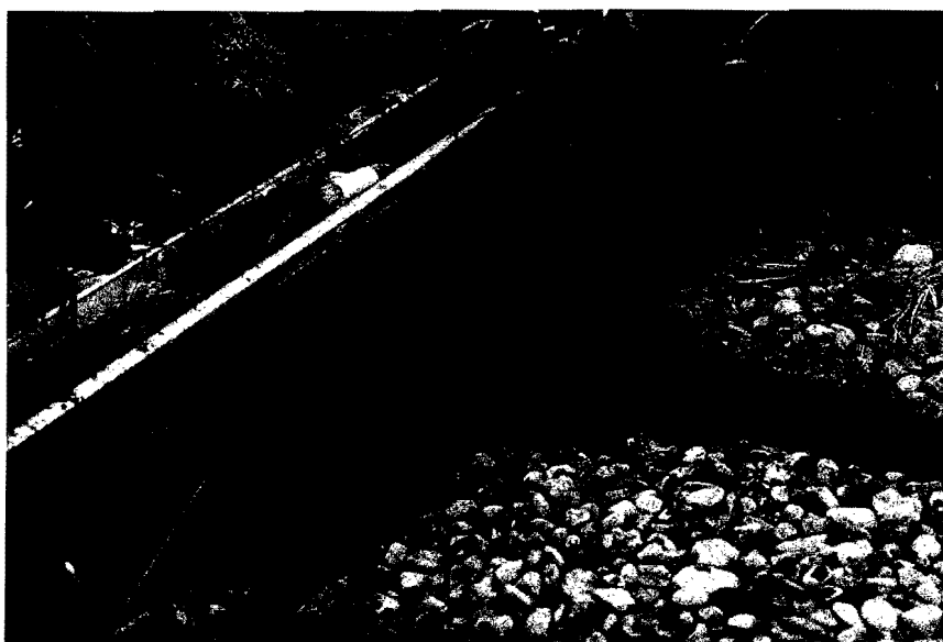
Figure 15. Solids deposition occurred both in the influent troughs and on the gravel layer.
