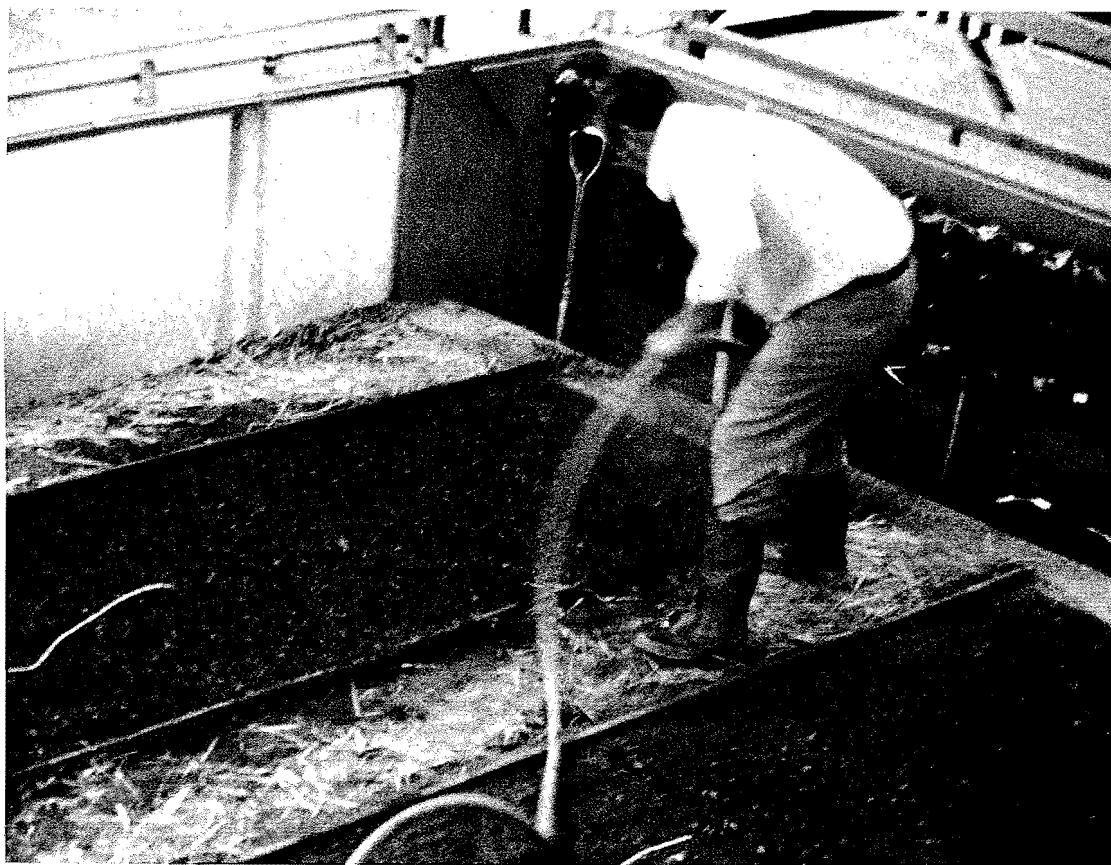
Figure 5. Applying mulch and seed with hydromulcher.
