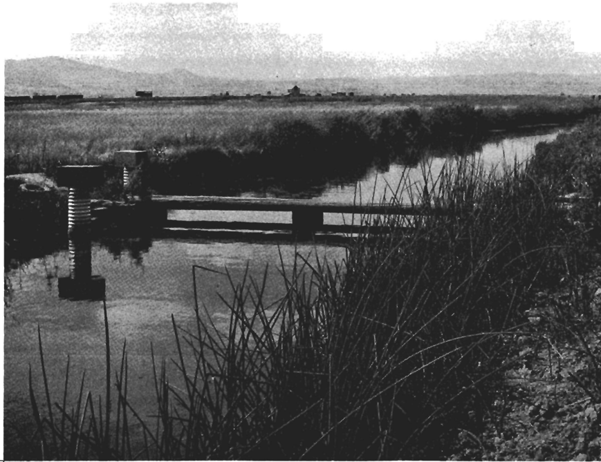
Figure 2. Downstream view of control structure.
