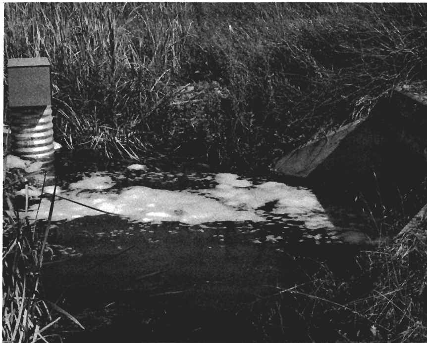
Figure 5. Looking at upstream side of box culvert.
