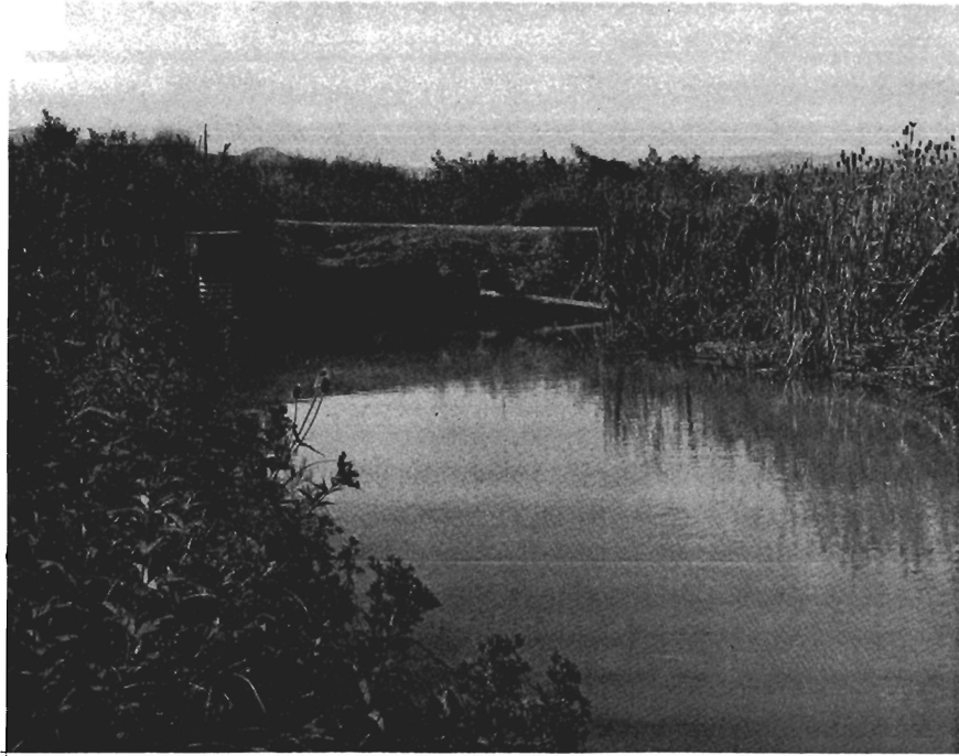
Figure 4. Looking at upstream side of corrugated culvert.
