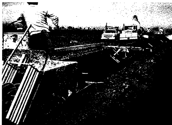
Concrete lining of a ditch in Imperial Valley, California.
