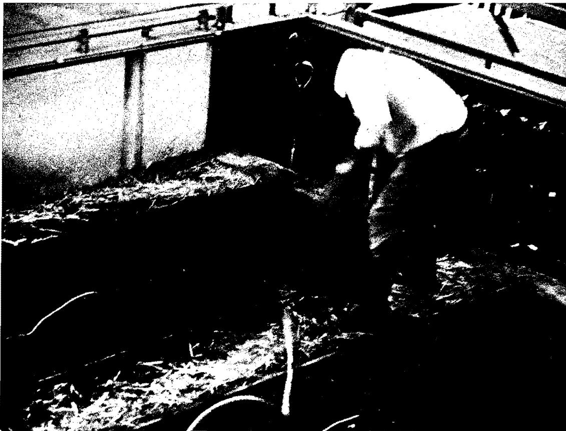
Figure 4. Applying mulch and seed with hydromulcher.
