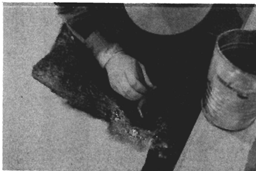
(c) Saturating the fiberglass mat with resin
