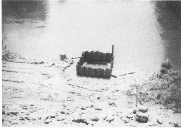
Figure A-10. Cofferdam
