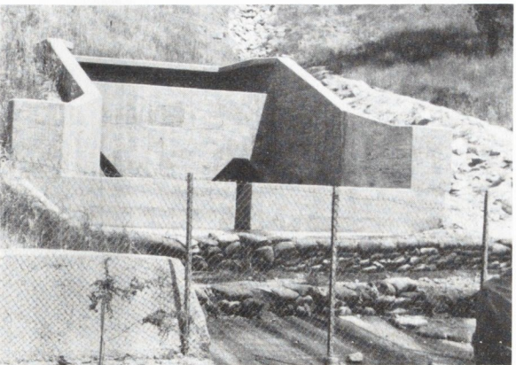
Figure A-21. Energy Dissipators
