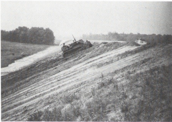
Figure A-57. Slope Grooming
