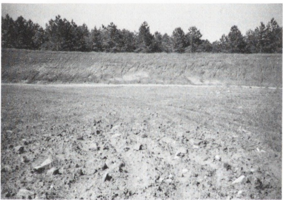
Figure A-45. Roughened Surface
