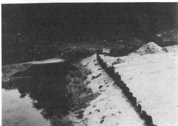
Figure A-54. Sheet Piling
