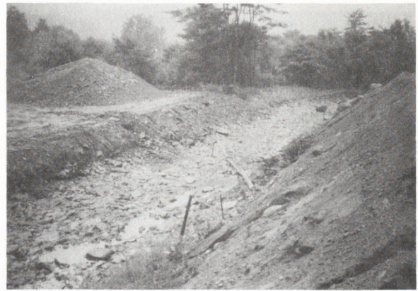
Temporary By-pass Channel
