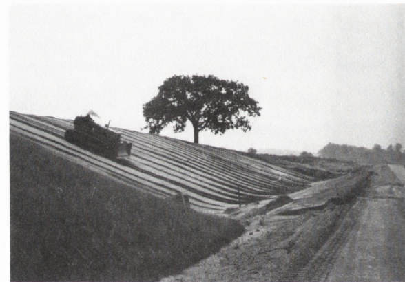
Figure A-52. Selective Grading & Shaping
