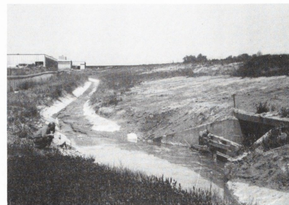
At Entrance to Culvert
