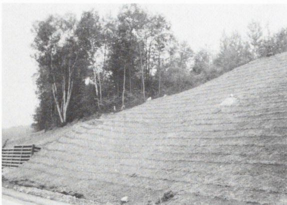
Stripping along Contours
