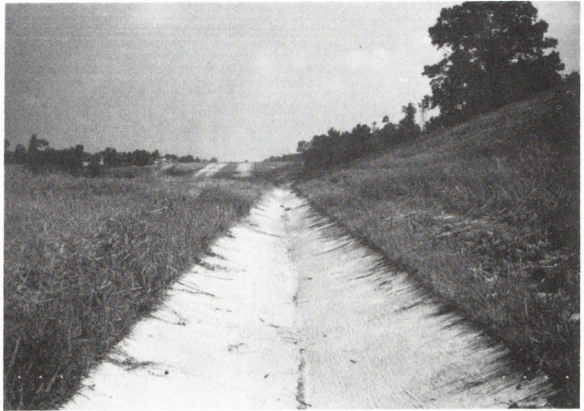
Figure A-72. Toe Drain Ditch
