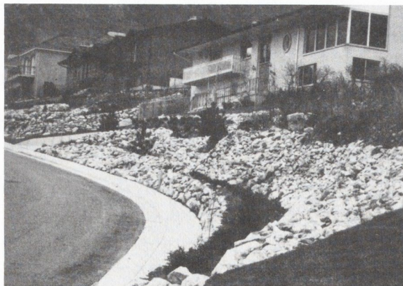
Figure A-69. Stabilizing With Rock
