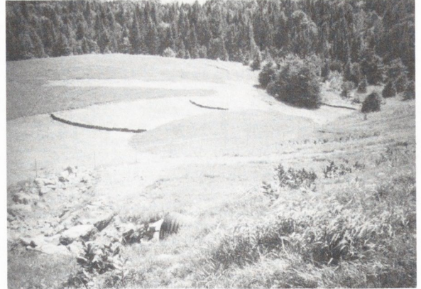
Figure A-22. Erosion Stops
