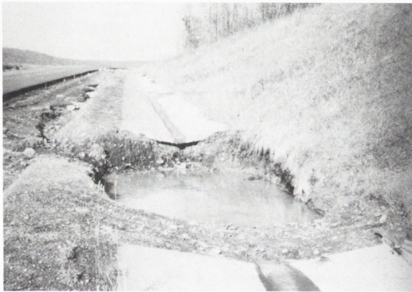
In Toe Drain
