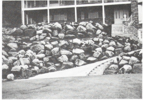
Figure A-69. Stabilizing With Rock (continued)
