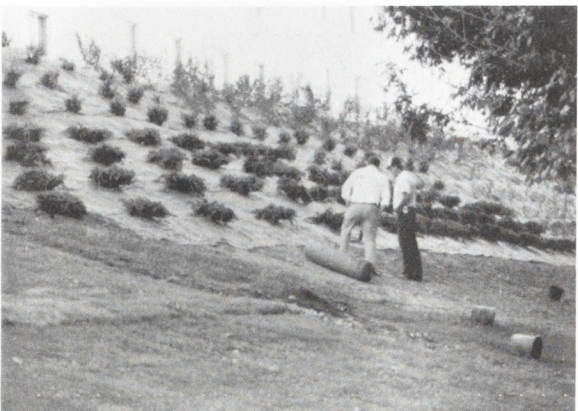
Jute and Sod
