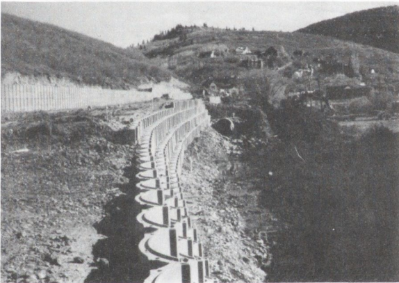
Figure A-42. Reinforced Earth Retaining Walls
