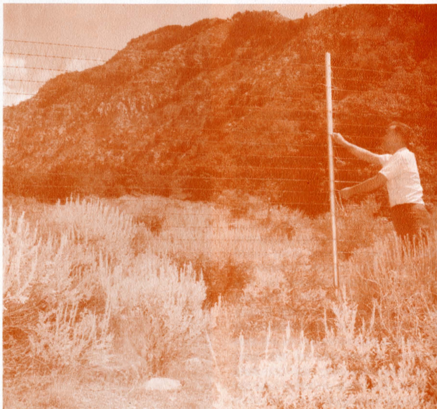
Figure 6. Where deer are plentiful and orchards are extensive, deer often feed on the trees during the winter. One way to prevent this is the construction of deer fences. This section of deer fence extends across the mouth of Dry Canyon in the vicinity of Logan, Utah.
