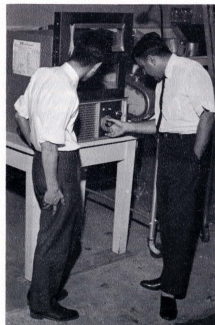
Figure 4. This microwave oven was used in dehydration studies.
