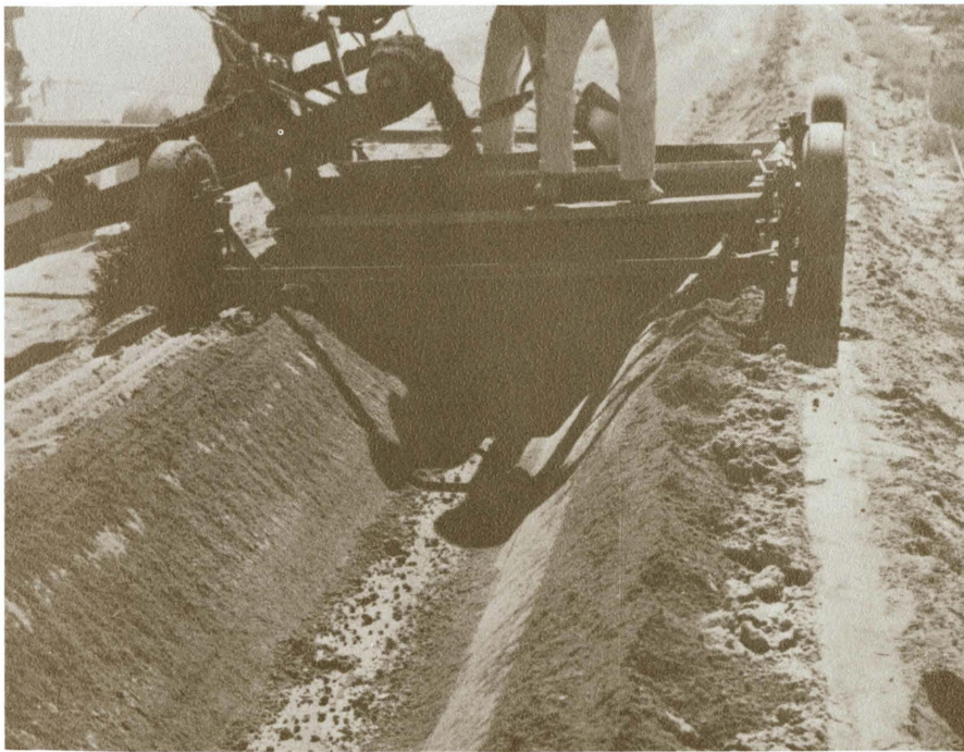
Figure 5. Spreader box consisting of a hopper and screed mounted on an adjustable frame carried on rubber-tired wheels.
