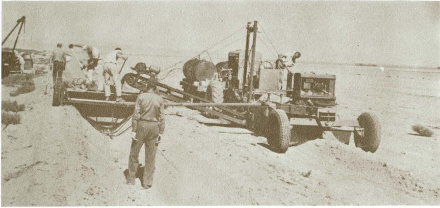
Figure 3. Wood Roadmixer assembly and spreader box mixing and placing soil-cement.
