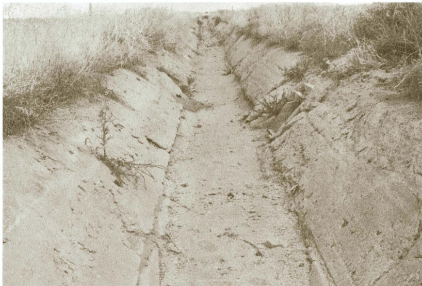
Figure 7. Condition of standard soil-cement lining with cement content of 5.2 percent on September 24, 1967—11 years after installation.
