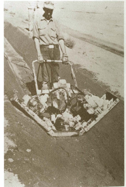
Figure 6. Jackson vibrator compacting soil-cement lining placed by spreader box.
