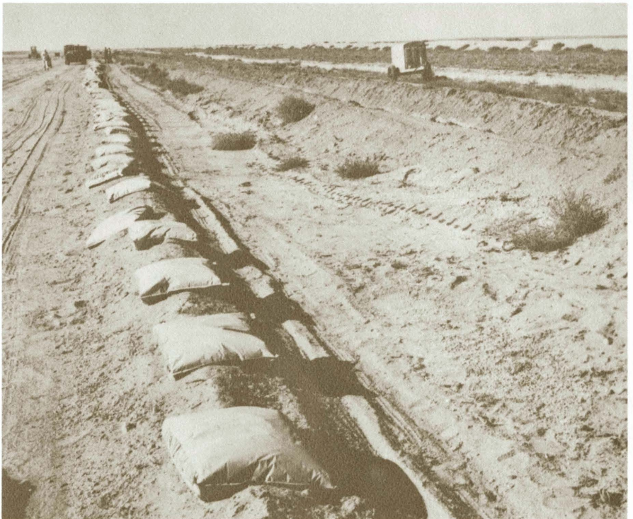
Figure 2. Cement bags spotted on windrow at proper spacing before being spread.
