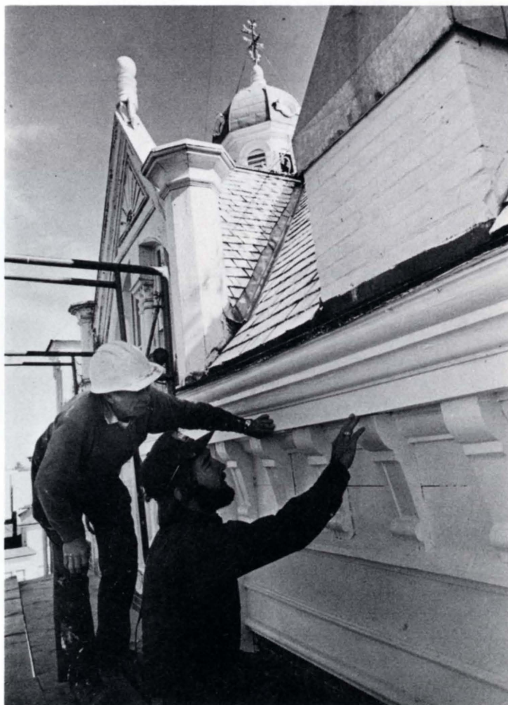
Workmen giving a facelift to the Beaver Courthouse.
