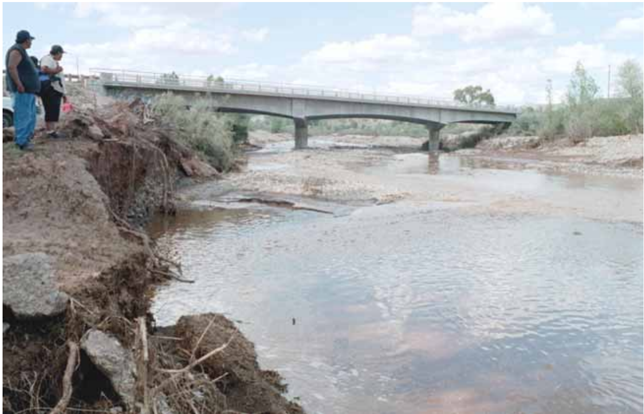
Figure 4: Staffers from the Watershed Program examine bank erosion below the lower bridge in Cibecue.
