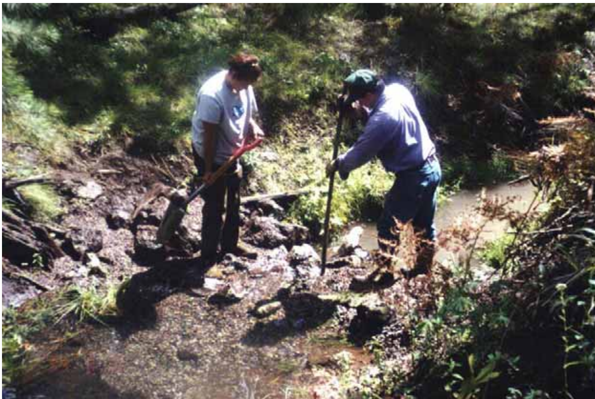
Figure 2: Co-author Candy Lupe and an outside researcher work together to install a riffle formation at a culturally important restoration site.
