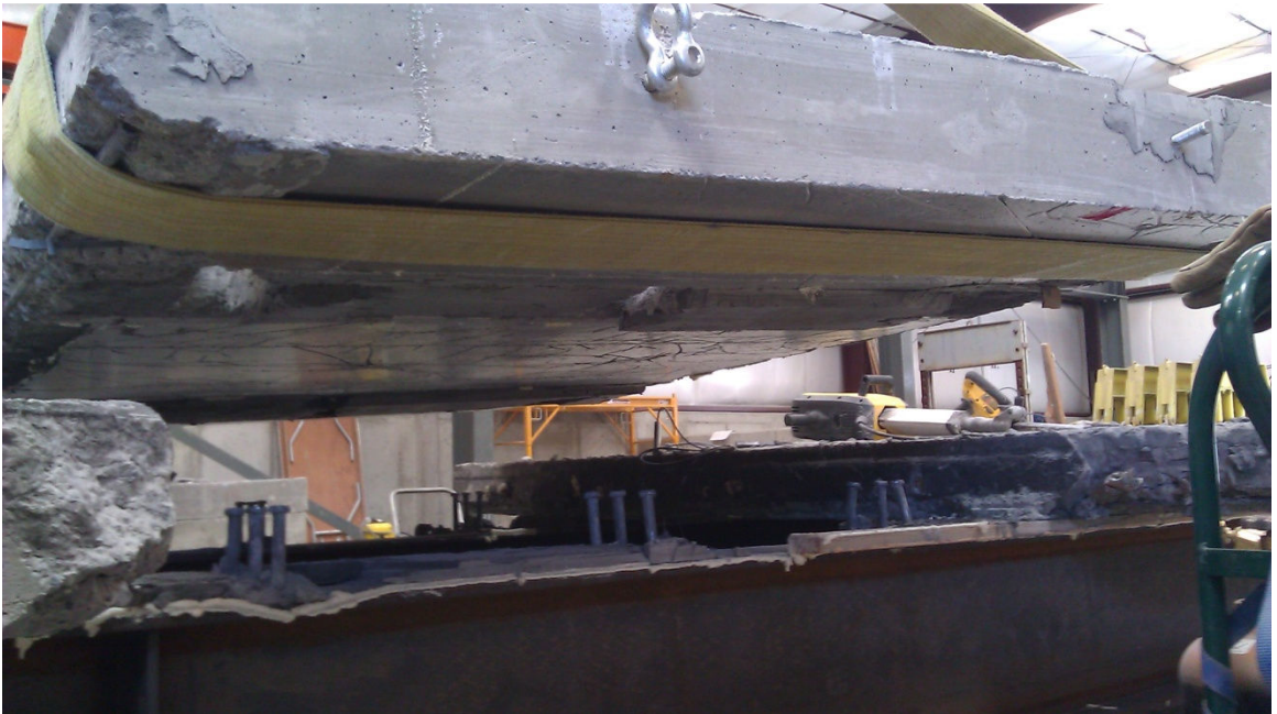
Fig. 16 Panel being replaced
