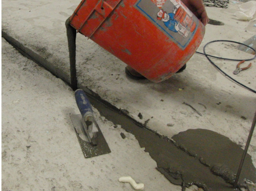
Fig. 17 Grouting of replaced joint.
