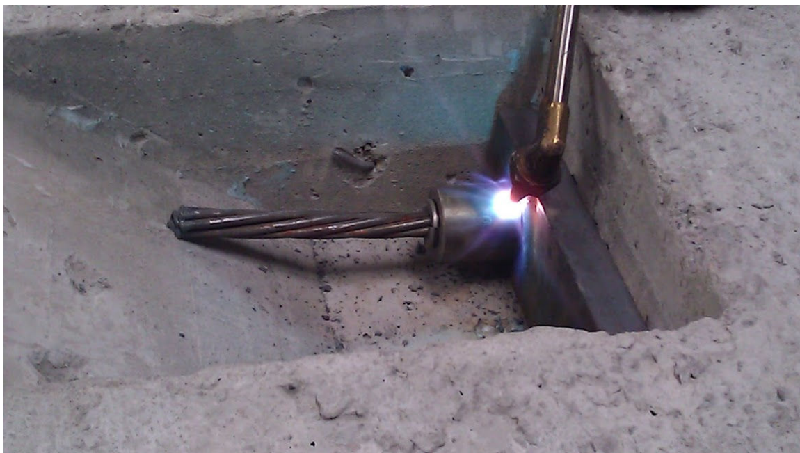
Fig. 12 Chuck and cable being removed
