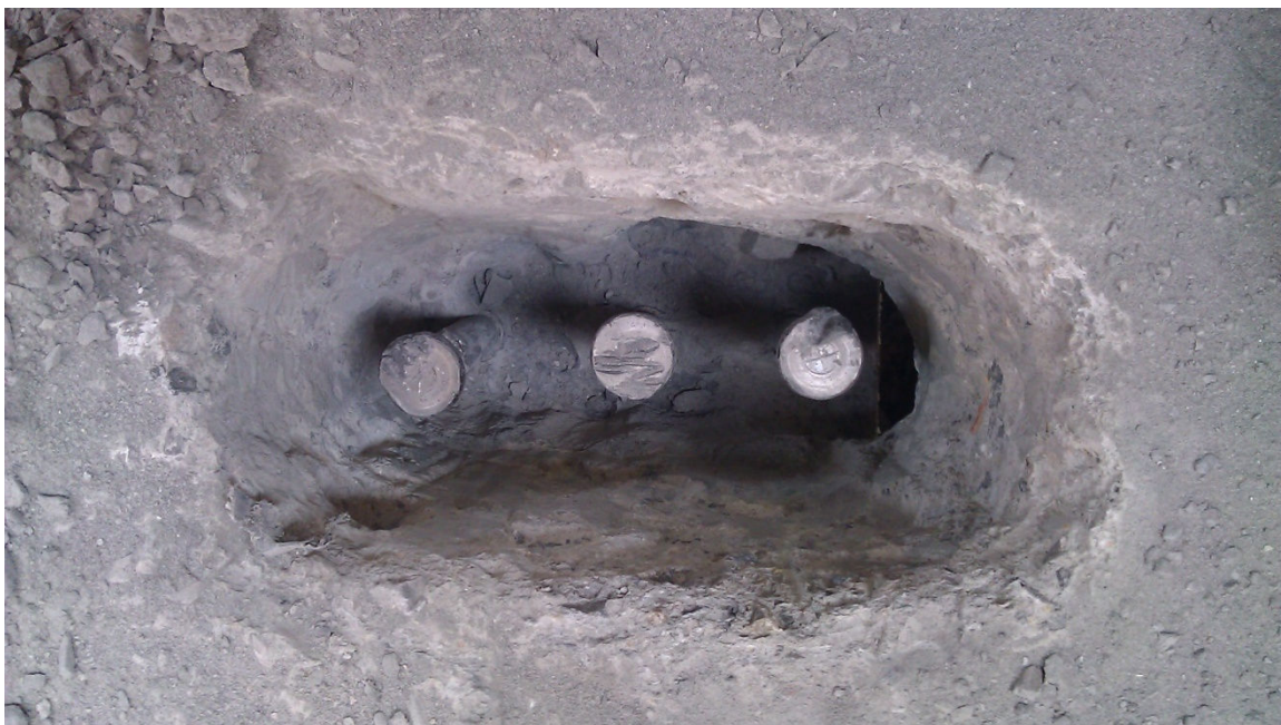
Fig. 14 Shear pocket after grout removal
