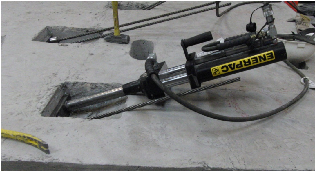
Fig. 18 Cables being stressed post panel replacement
