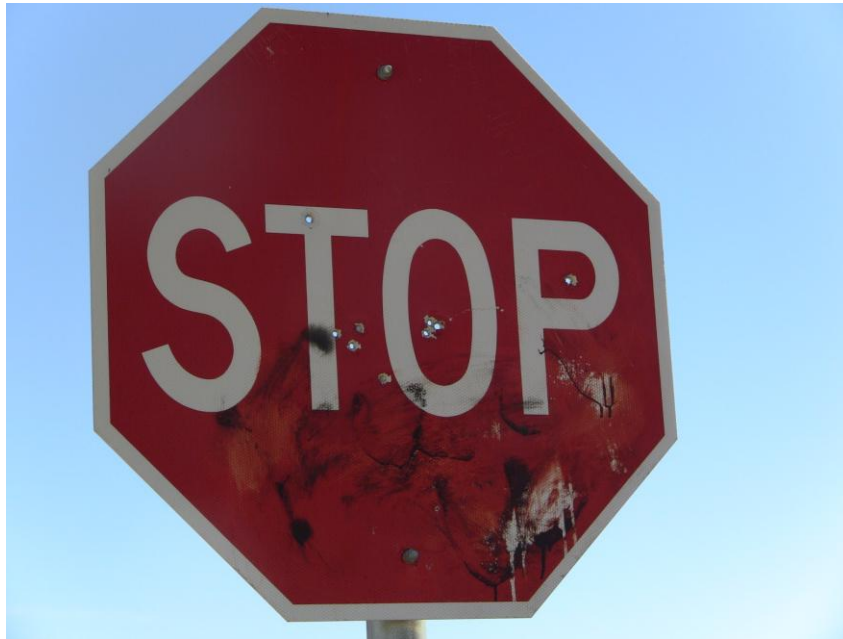
Figure 4.4 Graffiti cleaning attempt.
