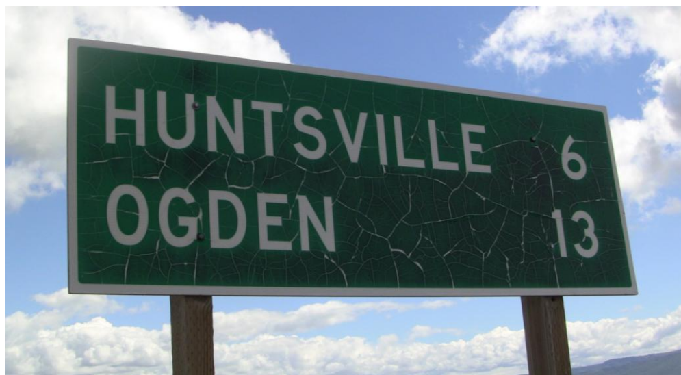
Figure 4.7 Type IX sheeting overlay failure.
