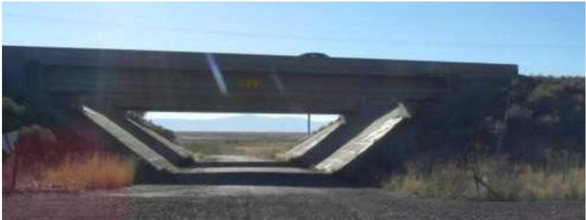
Figure 22 – Utah Bridge part of Interstate-15 (I-15) over Cannery Road.
