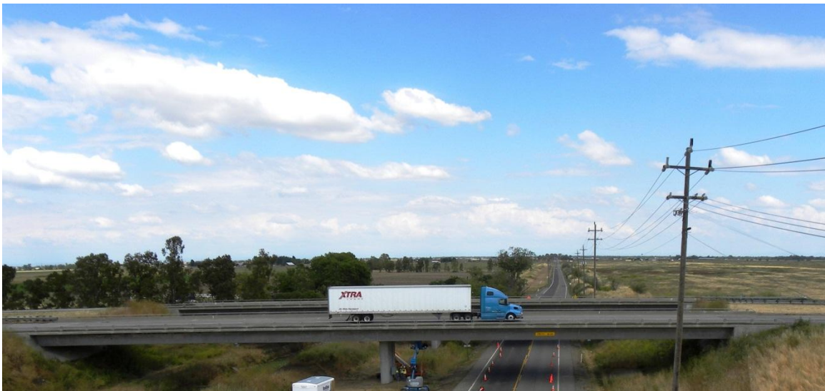
Figure 20 – California Bridge part of Interstate-5 (I-5) over Lambert Road.
