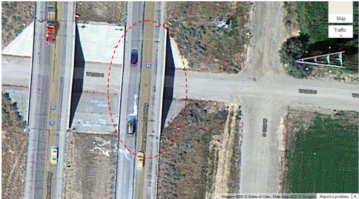
Figure 21 – Aerial view of the Utah Bridge.
