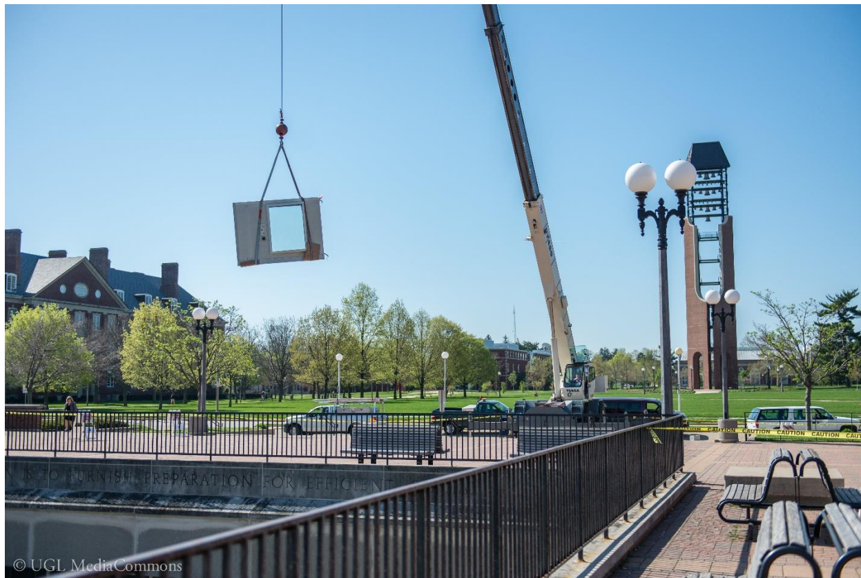
Image 5: Lowering the Audio Booth into the UGL
