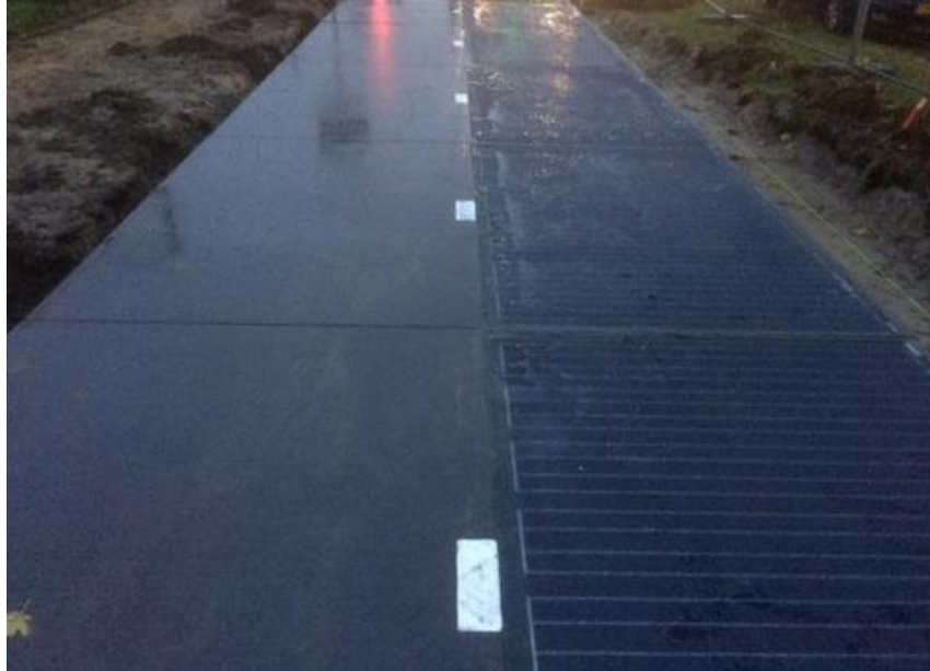
Figure 1-3: SolaRoad Pilot 2 (SolaRoad 2014)
