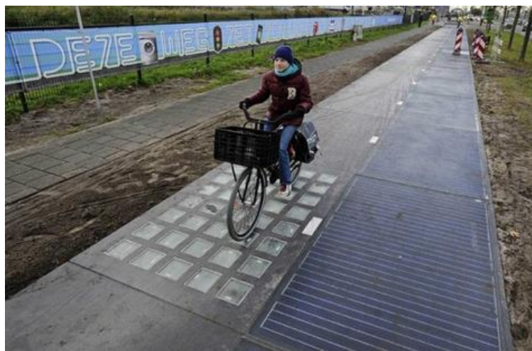
Figure 1-2: SolaRoad Pilot (SolaRoad 2014)
