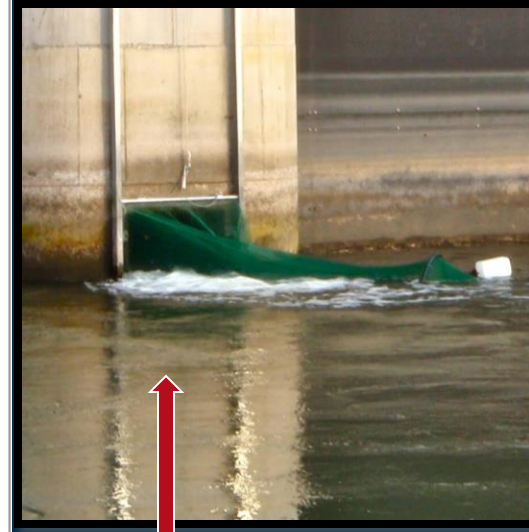
Small stow net at the exit of the eel-bypass
