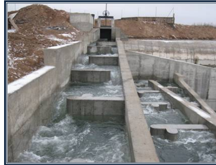
FISHWAY (SUMERGED NOTCH)
