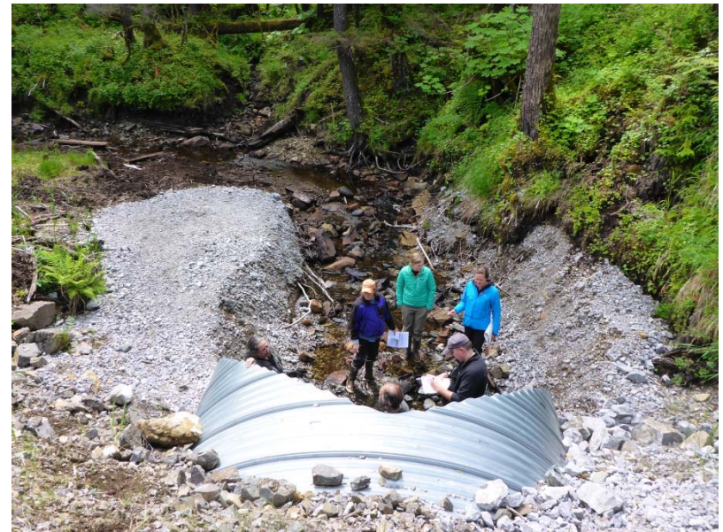
Bed material used to surcharge pipe with material
