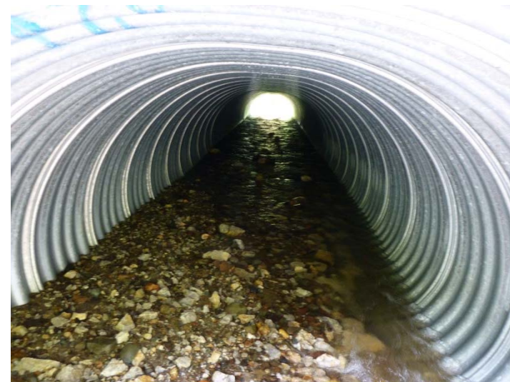
Embedded Structure Tongass N.F.
