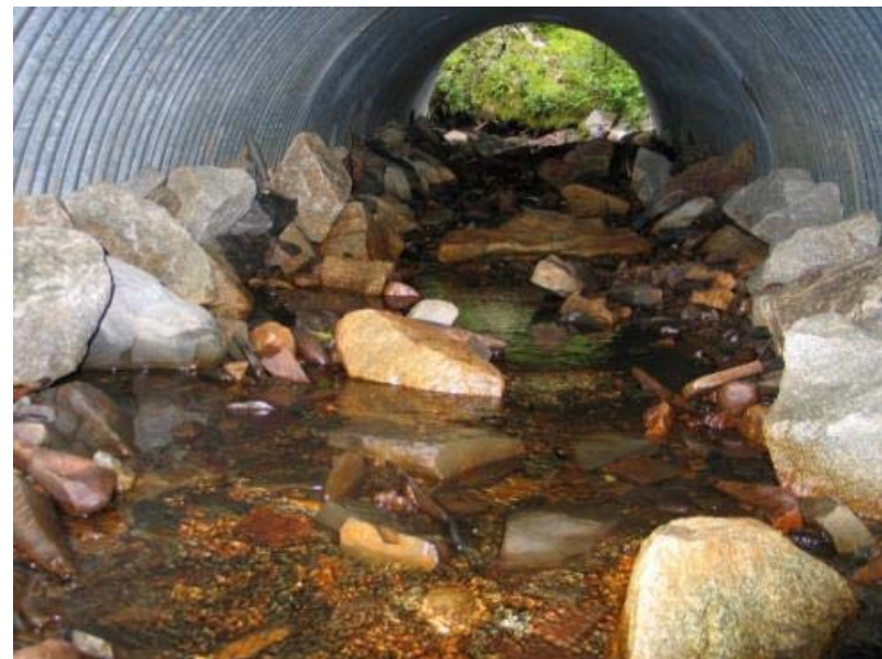
Stream Simulation Placed material AOP structure Tongass NF, Alaska
