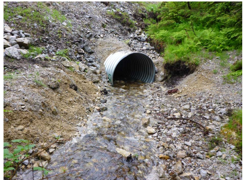
Overwide bank transition leads to long term aggradation
