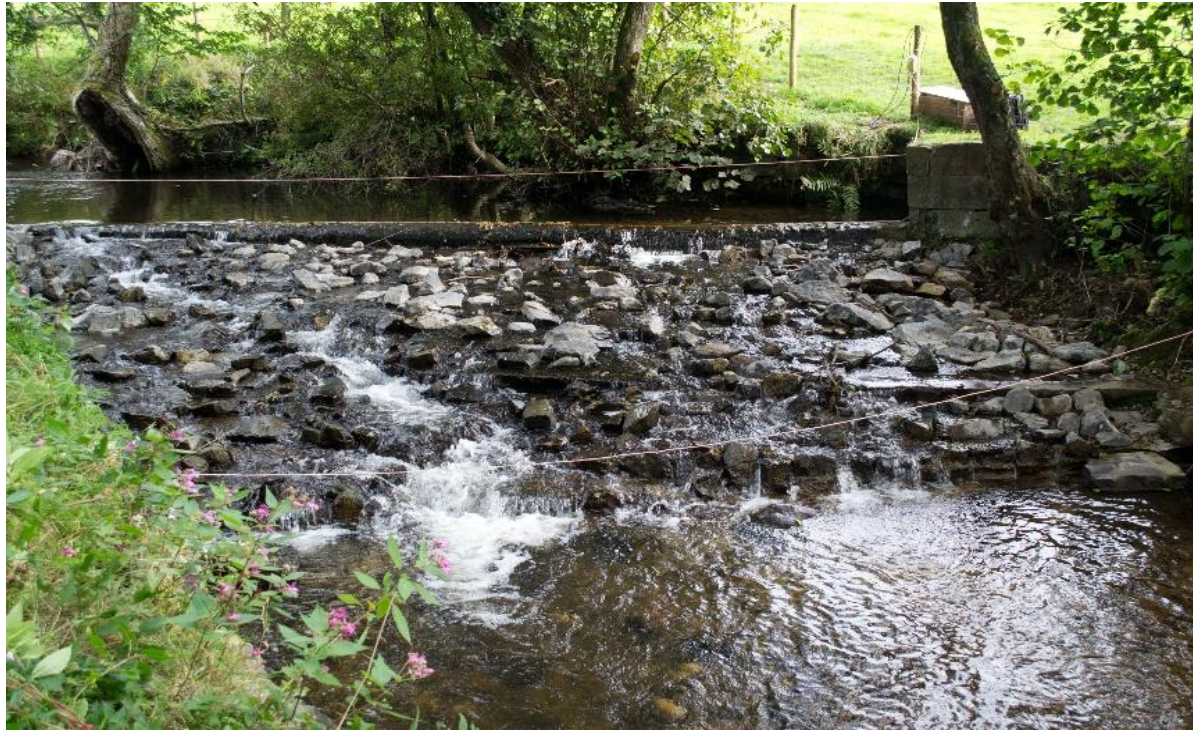
Embedded Rock Ramp (2014)
