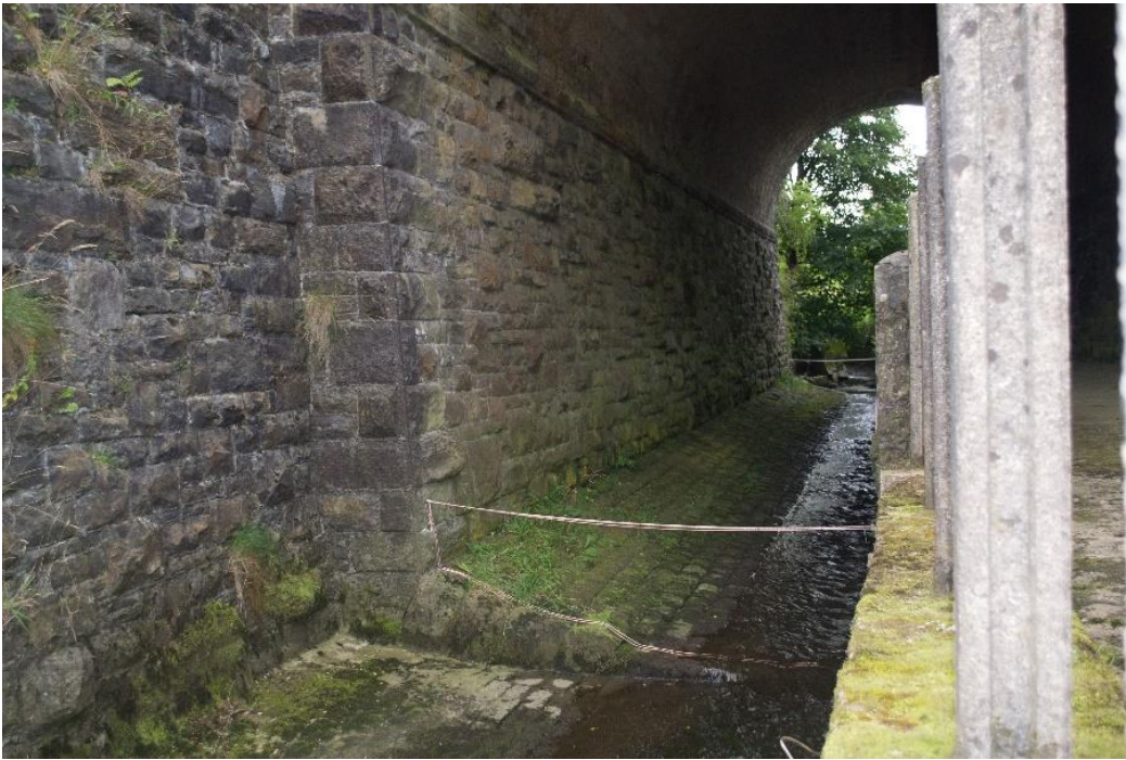
Culvert 1 (Control; 2013 and 2014) Length = 20 m, Slope = 4%, Mean V = 0.46 \text{ ms}^{-1}
