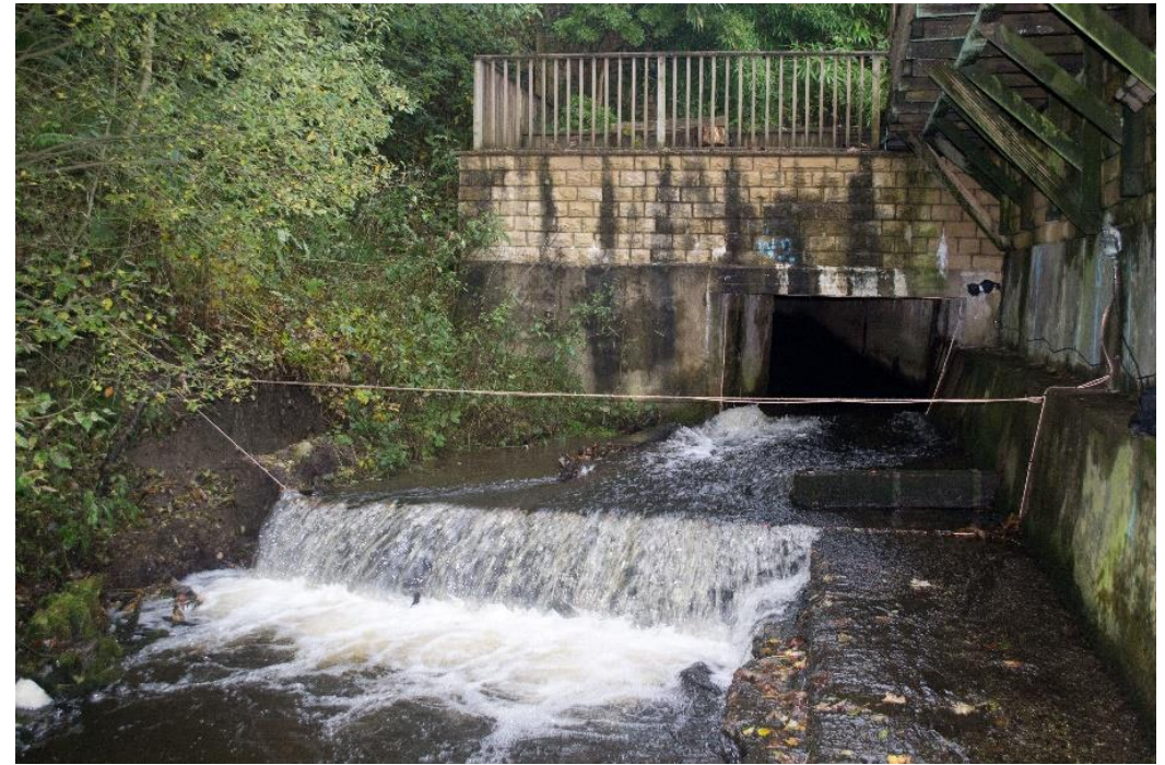
Culvert 2 (2013) Length = 70 m, Slope = 5.2%, Mean V = 2.32 \text{ ms}^{-1}
