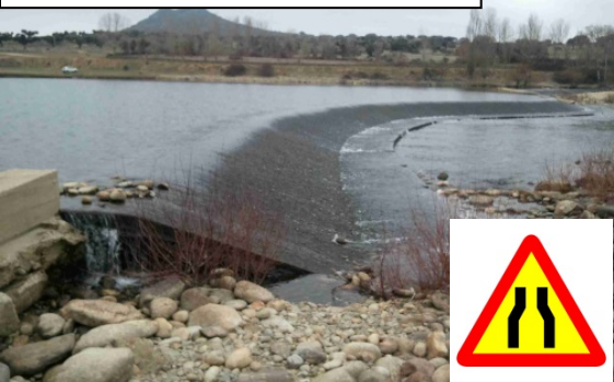
Weir in the reservoir tail
