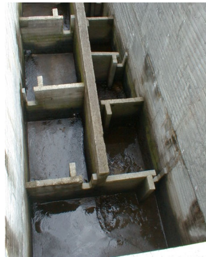
Pool-type fishway with cross-walls equipped with notches and bottom orifices in Nunes mini-hydroelectric plant
