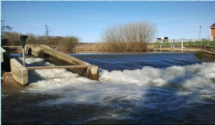
Buttercrambe weir at high flow (velocity over weir ca. 3 m/s), showing flow through Larinier pass
