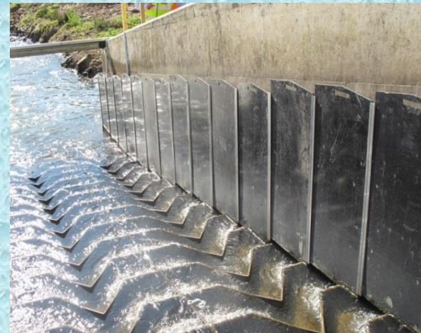
Dewatered pass with wall-mounted bossed tiles
