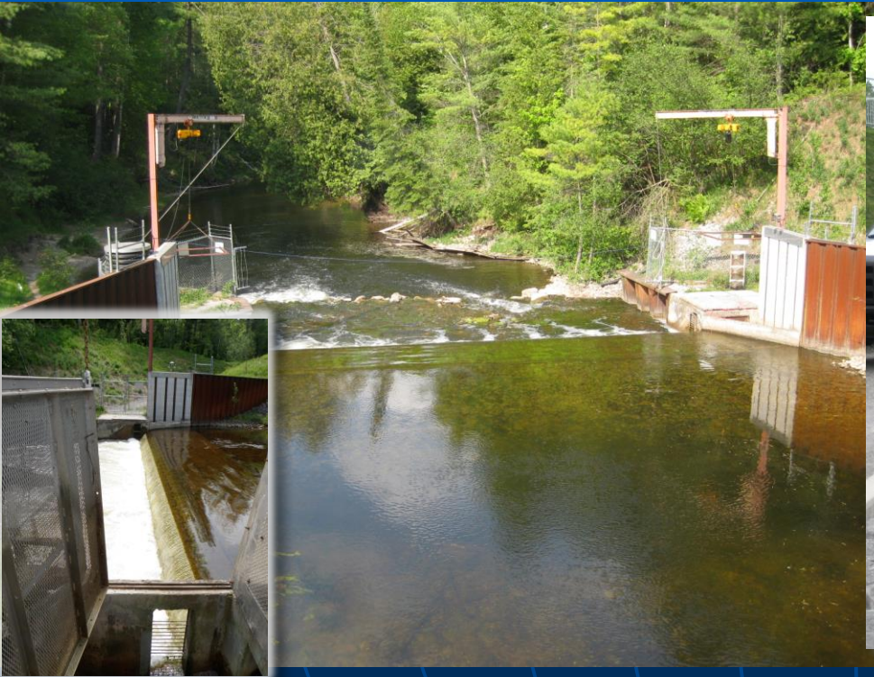
Ocqueoc River Weir: paired traps on opposite banks.
