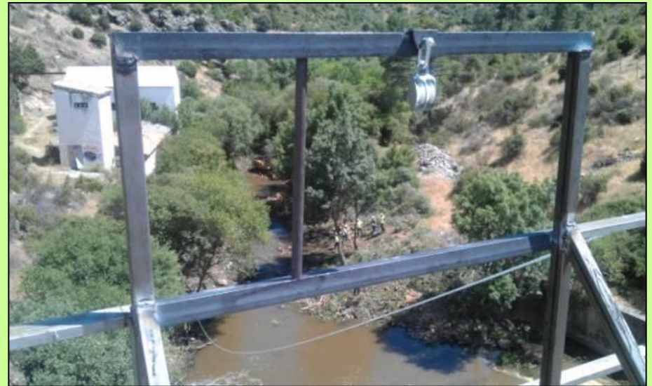
Zip-line for fish transfer from the empty reservoir to downstream
