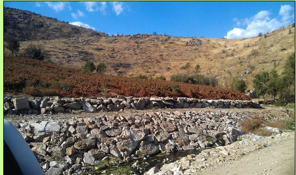
Sediments removed, stone protection and plantations
