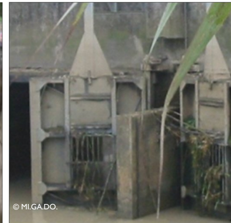
Tide gates with window present in the gates
