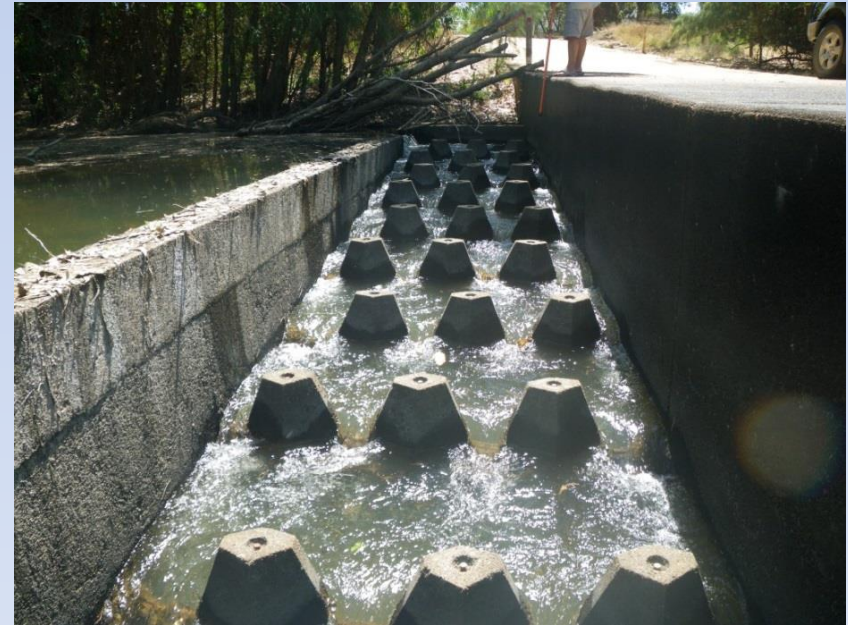
Pool-type fishways “cone fishway”
