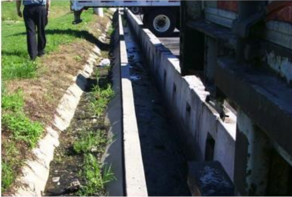
Figure 2.22: This photo shows the initial settling drain and vegetated filter strip used to treat the first flush during storm events (Department of Environmental Protection, 2006).
