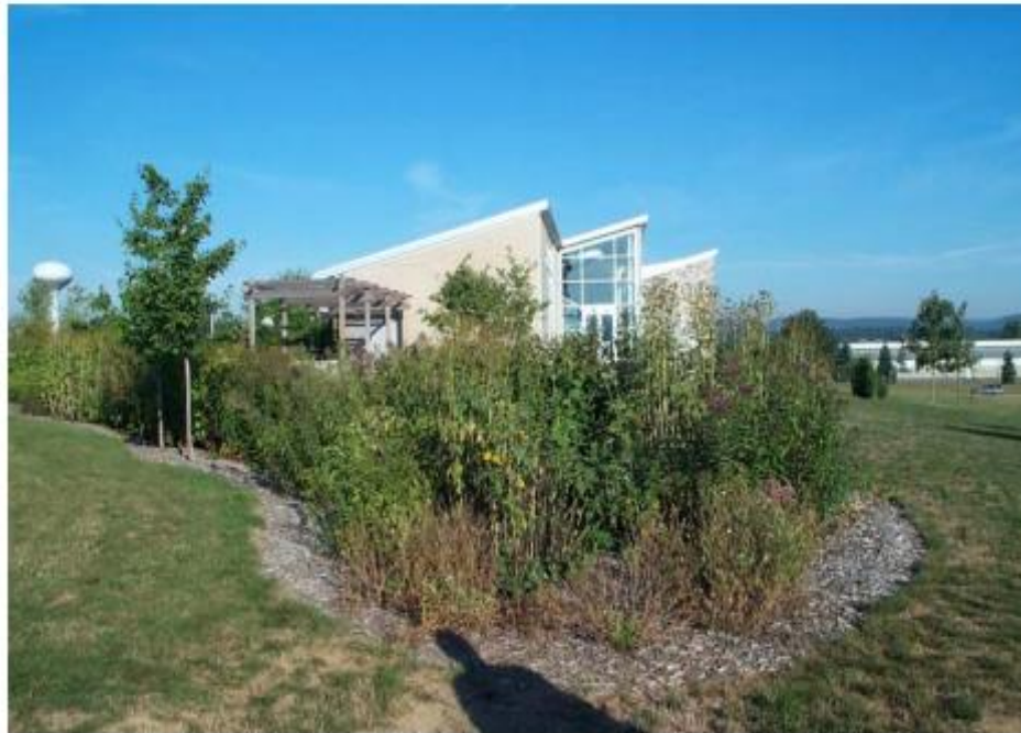
Figure 2.20: The Centre Visitor Center vegetated bioretention area (Department of Environmental Protection, 2006).
