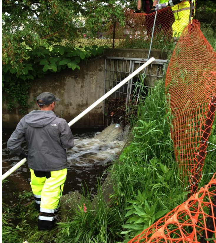
Figure 3.6: A second UMass Physical Plant team works to clean out debris and sediment blocking the outlet pipe at the west gate entrance to campus (photo credit: Nathan Frazee).
