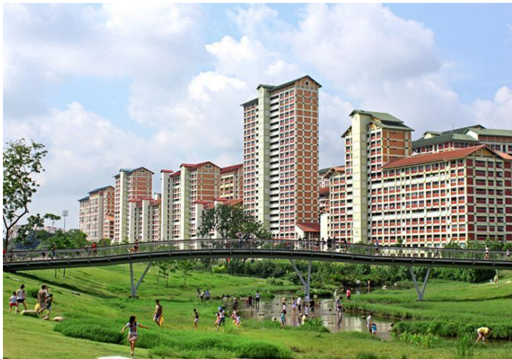
Figure 2.16: Before photo (left) of the utilitarian concrete channel in contrast with an after photo (right) of the naturalized stream with lush vegetation and resources for community engagement (Atelier Dreiseitl, 2015).
