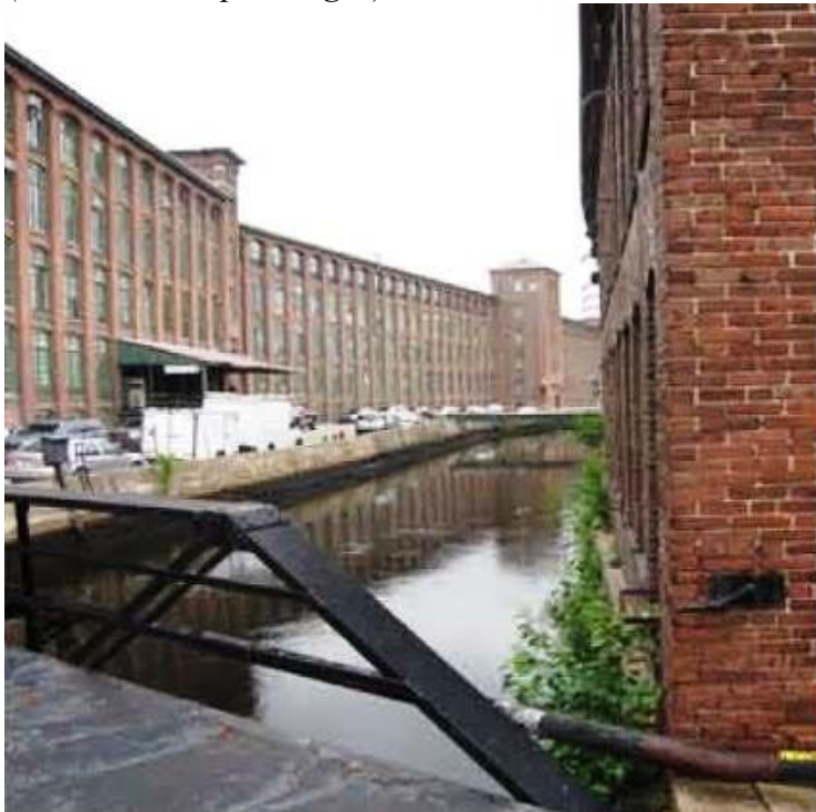
Figure 7. Cabotville Mill Complex (Source: Chicopeema.gov)
