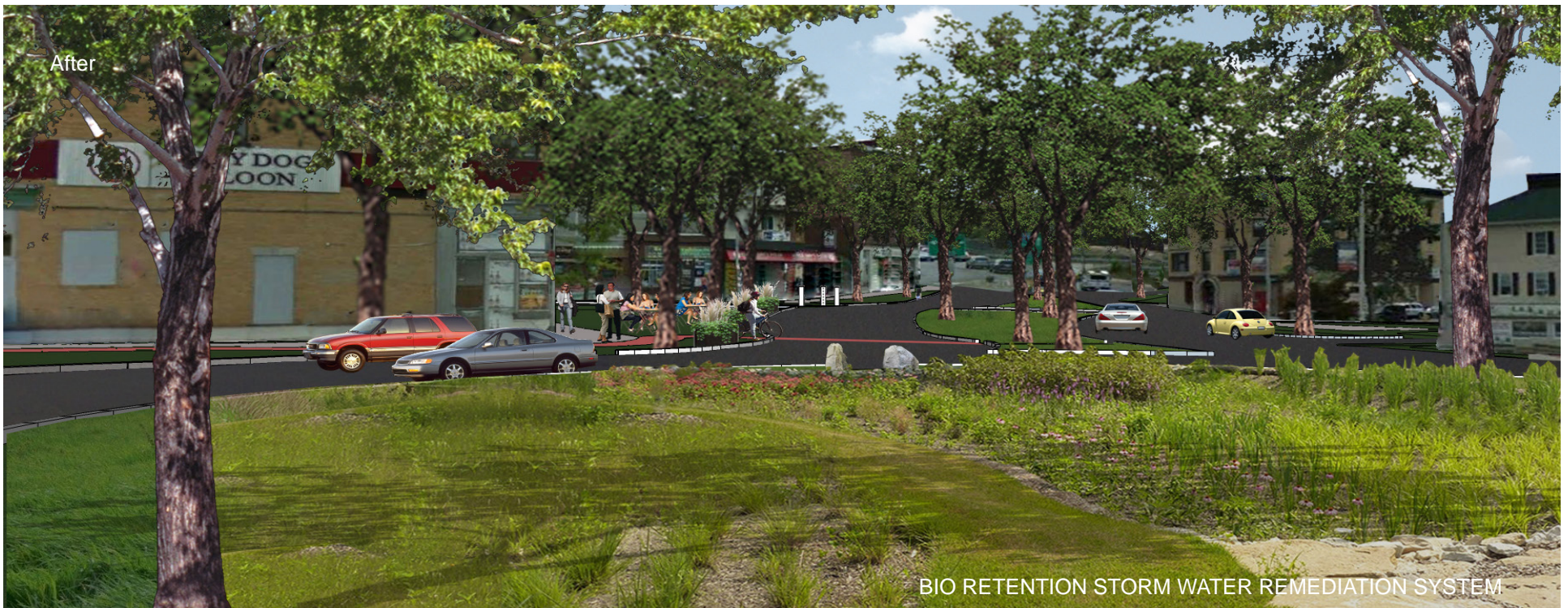
An after image showing the new green space created by implementing a traffic circle in this area. This new green space will become a designed Bioretention Storm Water Remediation/Infiltration System.
