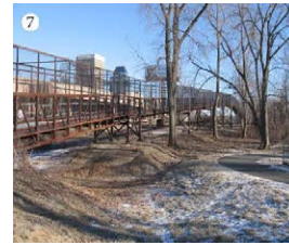
7. Curved topographic foot path and elevated steel bridge.
