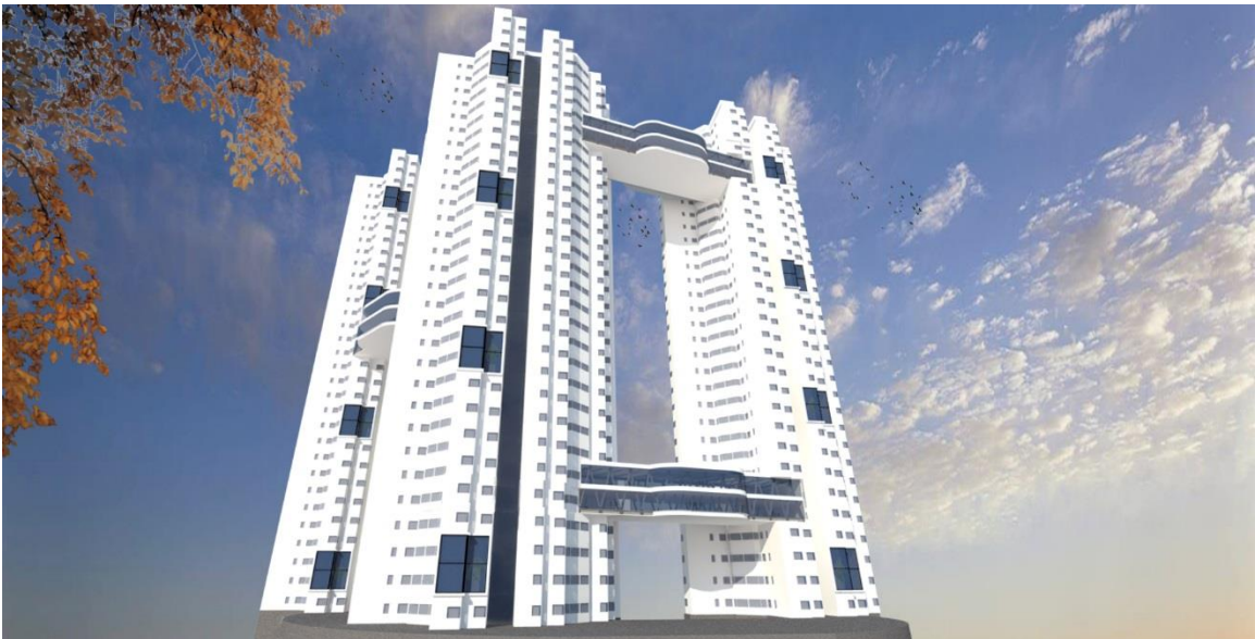
Figure 6.12 Perspective of the renovated project
