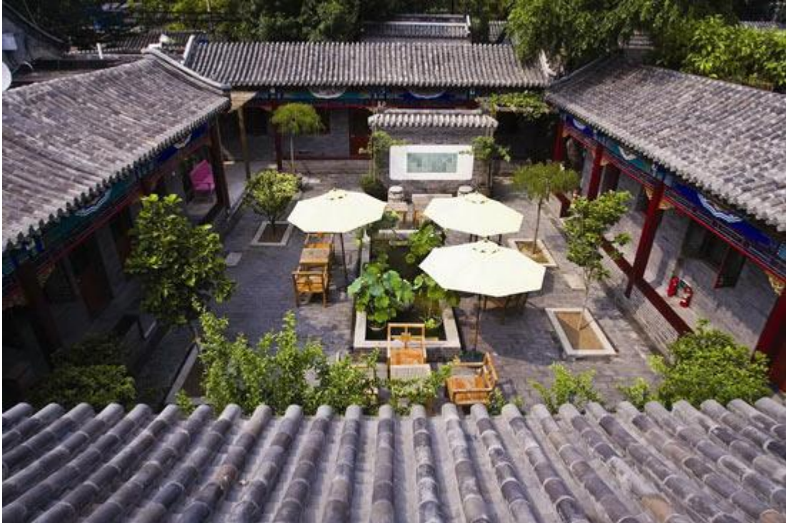
Figure 5.11 The second-step courtyard
