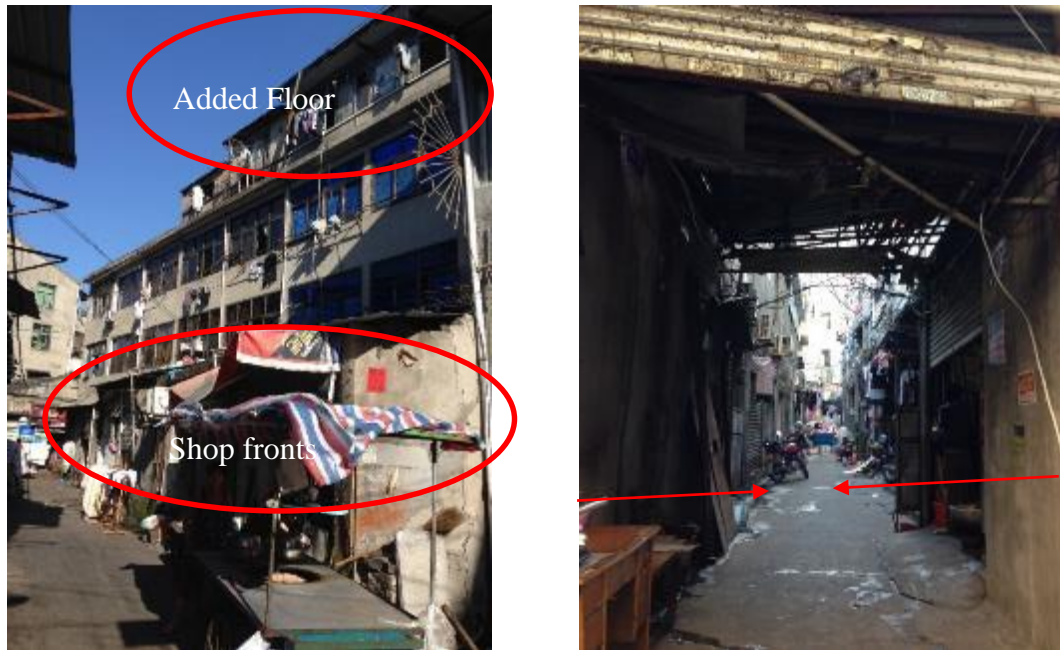
Figure 6.7 Illegal adherence VICs buildings in Jishi village
