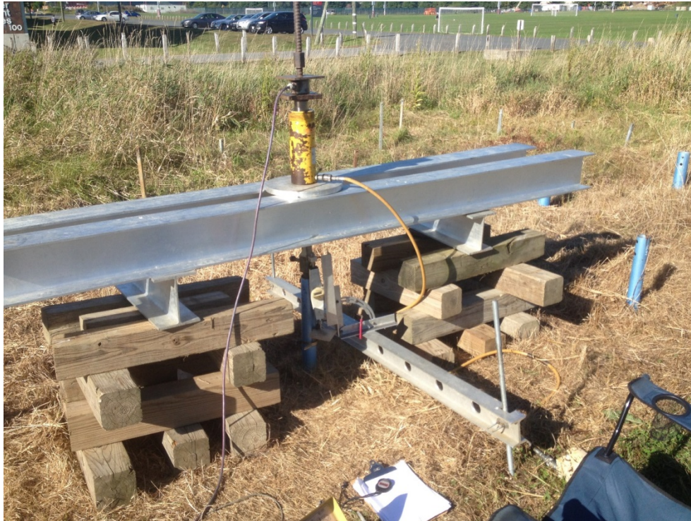
Figure 4.14 Typical Setup for Uplift Test of Helical Anchor at UMass-DOE Site
