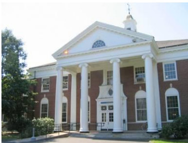
Goodell Building Storage – 7,300 sf
