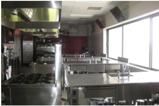
Instructional Kitchen– Campus Center
