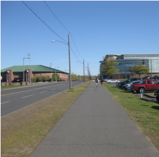
Excessive paved surfaces
