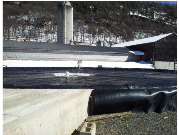
Picture 1: Barstow Digester Manure Tank
