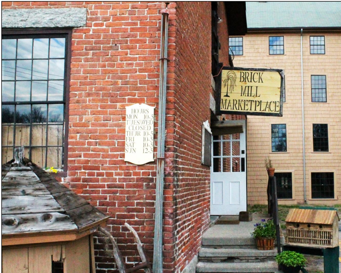
Figure 8. The sole tenant in the SWM is an antique shop. The remaining commercial space in the complex is still under construction.
