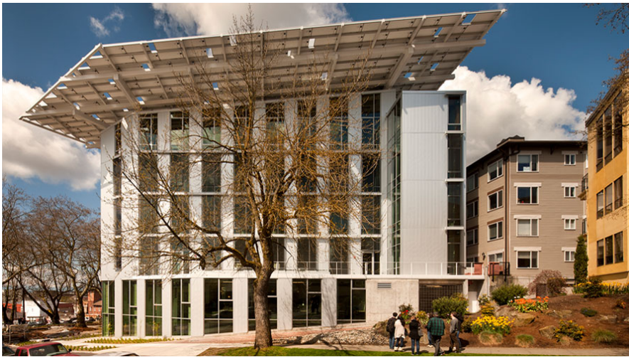
Figure 4: Bullitt Center Seattle, WA Miller Hull
