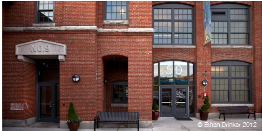
Figure 10: Union Crossing Building 9 Lawrence, MA Coldham and Hartman
